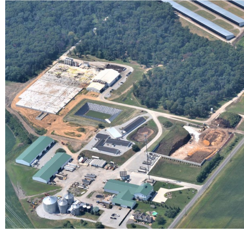
Conversion of waste to power and heat from RNG/biomethan - BioTown Biogas, Inc.
